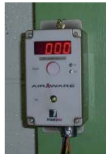
Fig. 1: The "AirAware" monitor, suitable for installation in a garage, detects "trigger" CO levels and sounds an alarm.
